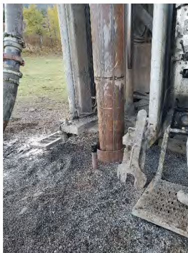
COMPLETED CAISSON. DRILLING \varnothing 12" SURFACE CASING
