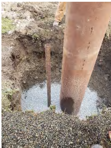
\varnothing 16" CAISSON, \varnothing 2" STANDPIPE AND ENGINEERED FILL
